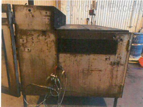
SIDE and REAR VIEW
